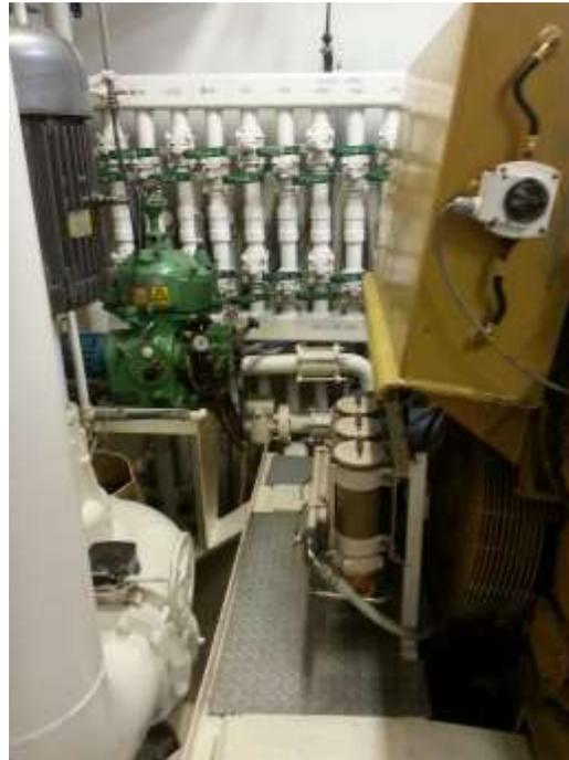
Westfalia fuel centrifuge (l), fuel manifold and day tank(c), 3508 Cat main and Racor water separators(r)
