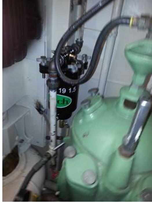
Fitch FHD5 used to pre-treat fuel in 4,000 gallon day tank (max 300 gph)
