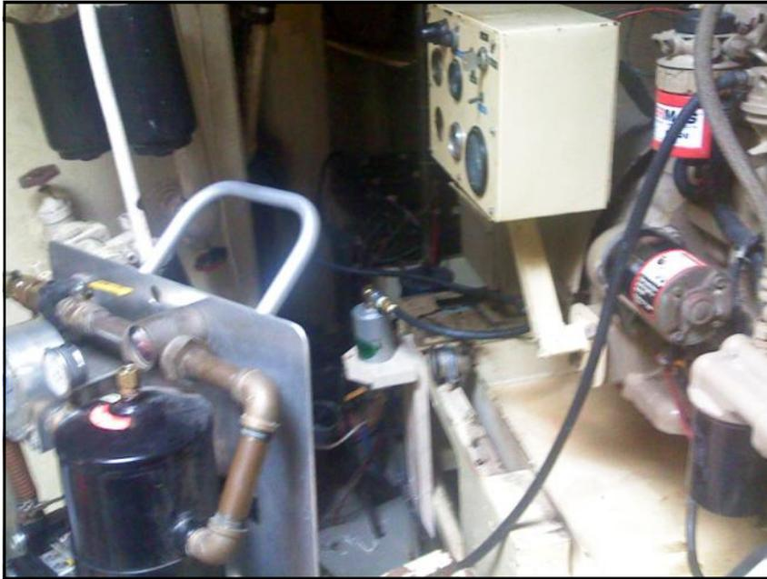
John Deere engine used with 100 Kw generator with Fitch Heavy-Duty unit mounted on wooden support bracket. Close up of installation below.
